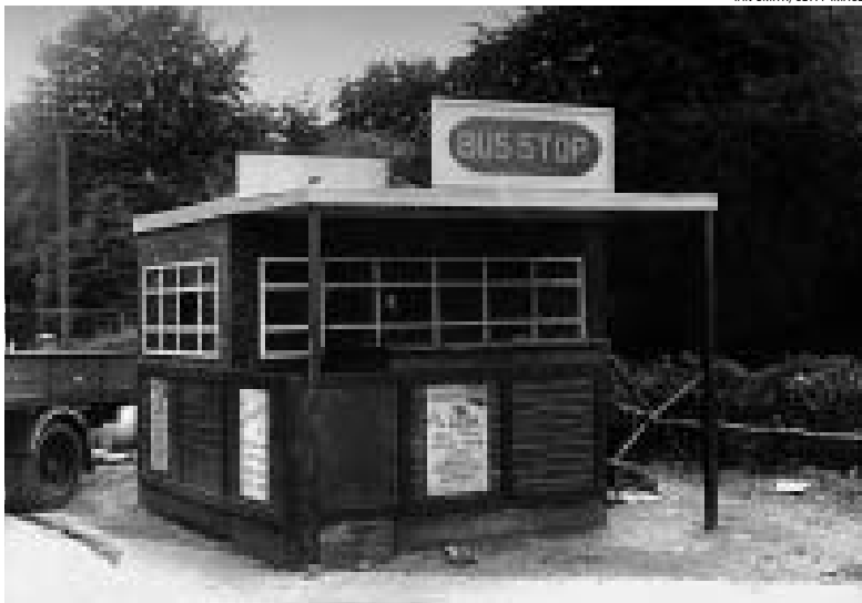
Do not alight here: this pillbox was disguised as a bus shelter in 1944
